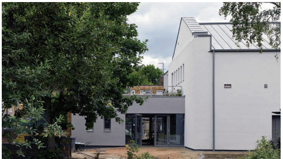
Above: Beneath all the polystyrene and render sits a 1890s generating station. There was little dismantling.
