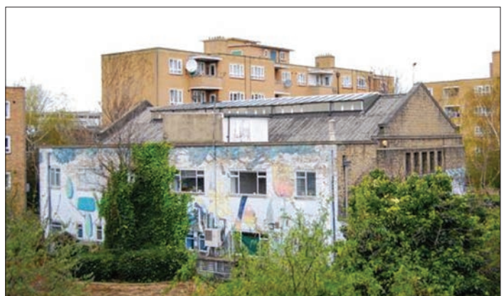
Right: The Mayville Community Centre prior to the refurbishment: leaky, energy hungry, and run-down – but still playing a vital role for the local community.
